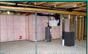
The basement has been studded, insulated, wired and ready for drywall. The rough-in for a basement washroom has also been installed
